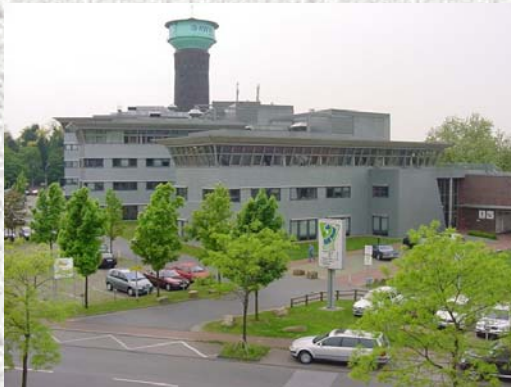
ACCESS Systems Europe (Oberhausen, Germany)
